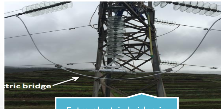
Electric continuity when line repowering required
